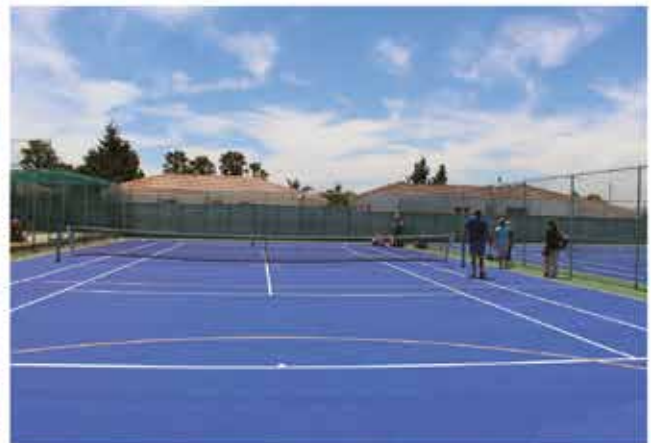
SENIOR PRIMARY Tennis courts resurfaced
