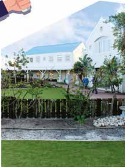
BLOUBERG PREPARATORY Installation of artificial turf
