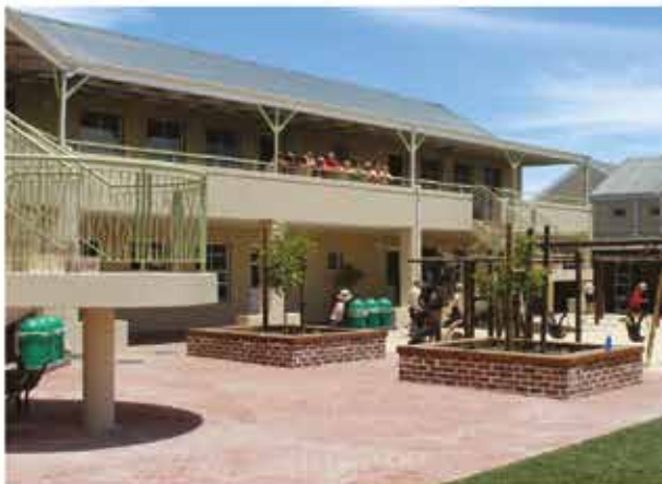
SUNNINGDALE PREPARATORY New Grade 3 classrooms completed
