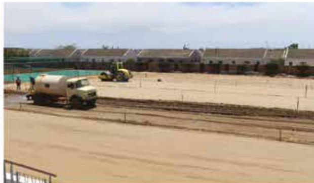
HIGH SCHOOL Construction of the astroturf commences
