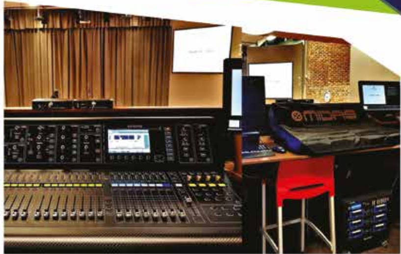
THEATRE@ELKANAH Technical sound equipment upgrade
